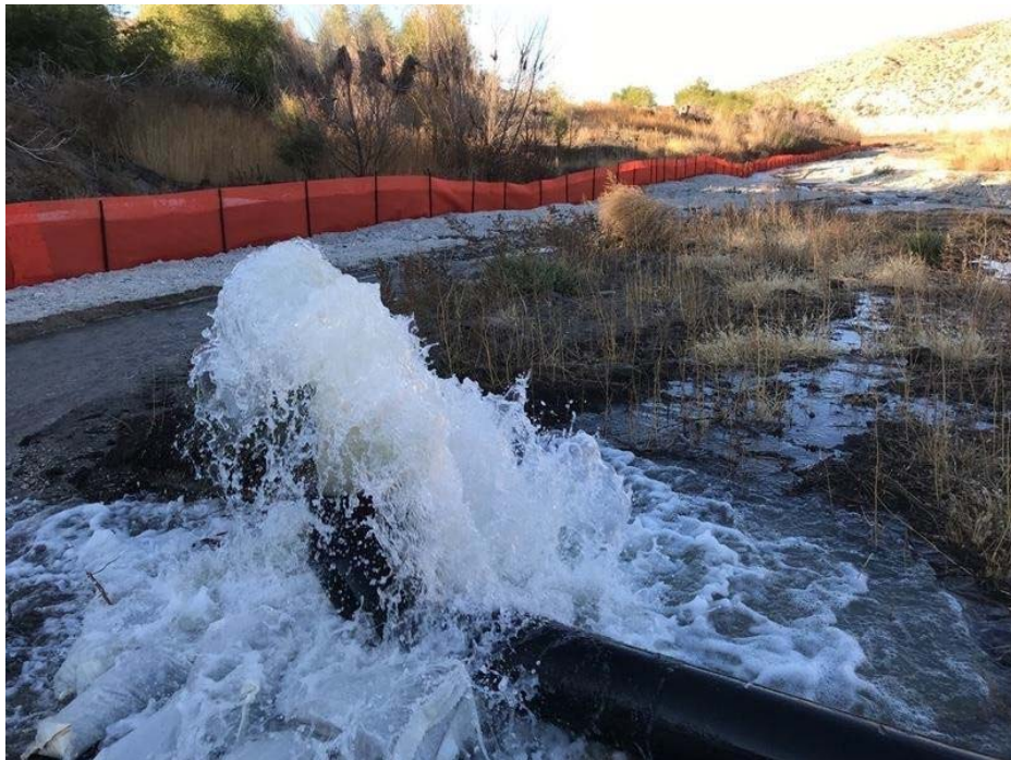
Photo 2. Dewatering well outflow pipe (November 6, 2018)
