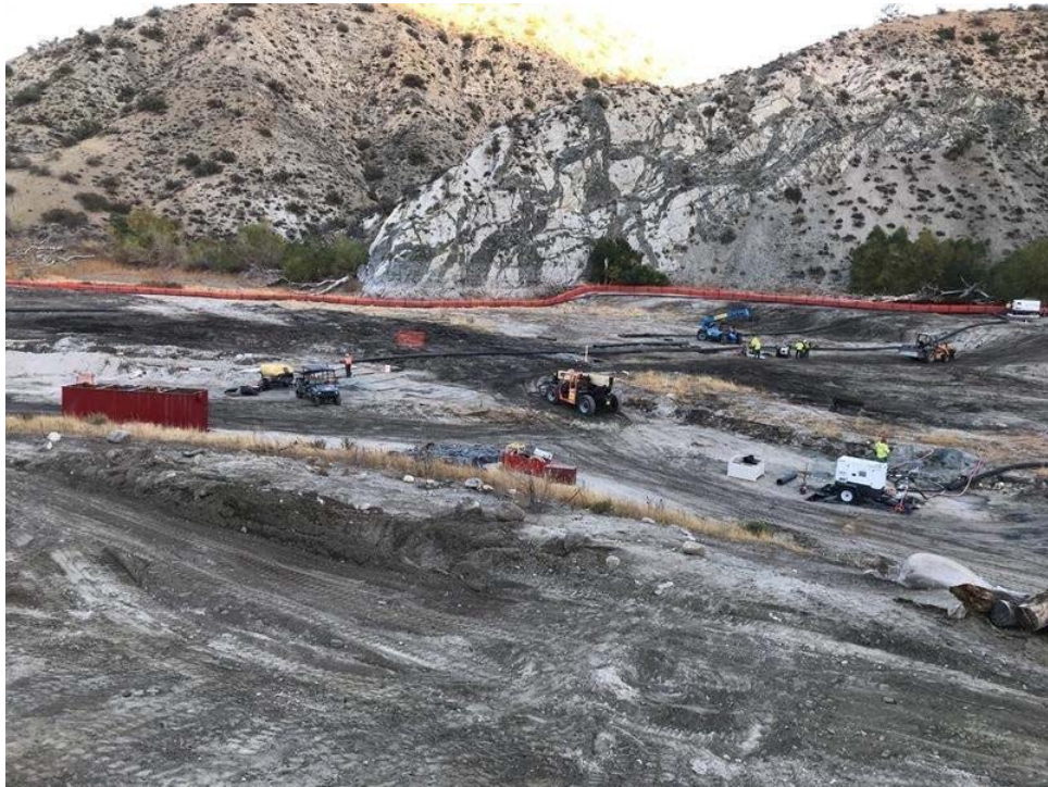
Photo 1. Dewatering wells operating at Rocky Point (November 5, 2018).
