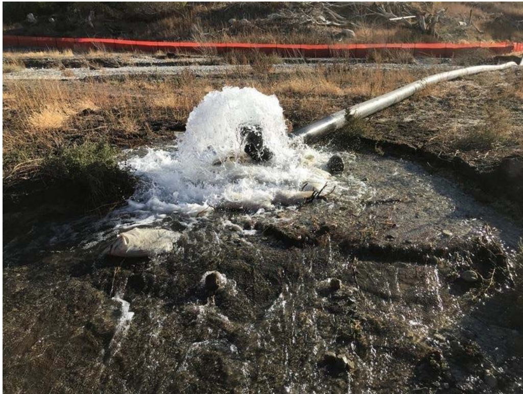
Photo 3. Dewatering well outflow pipe (November 9, 2018).
