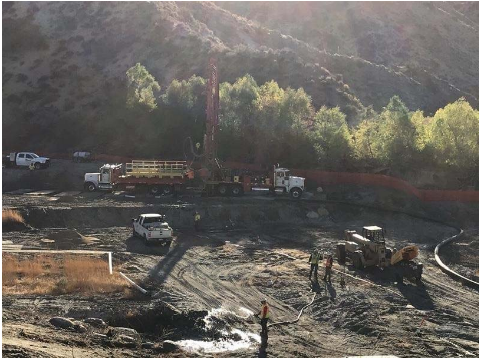
Photo 2. Drilling a dewatering well (October 31, 2018).
