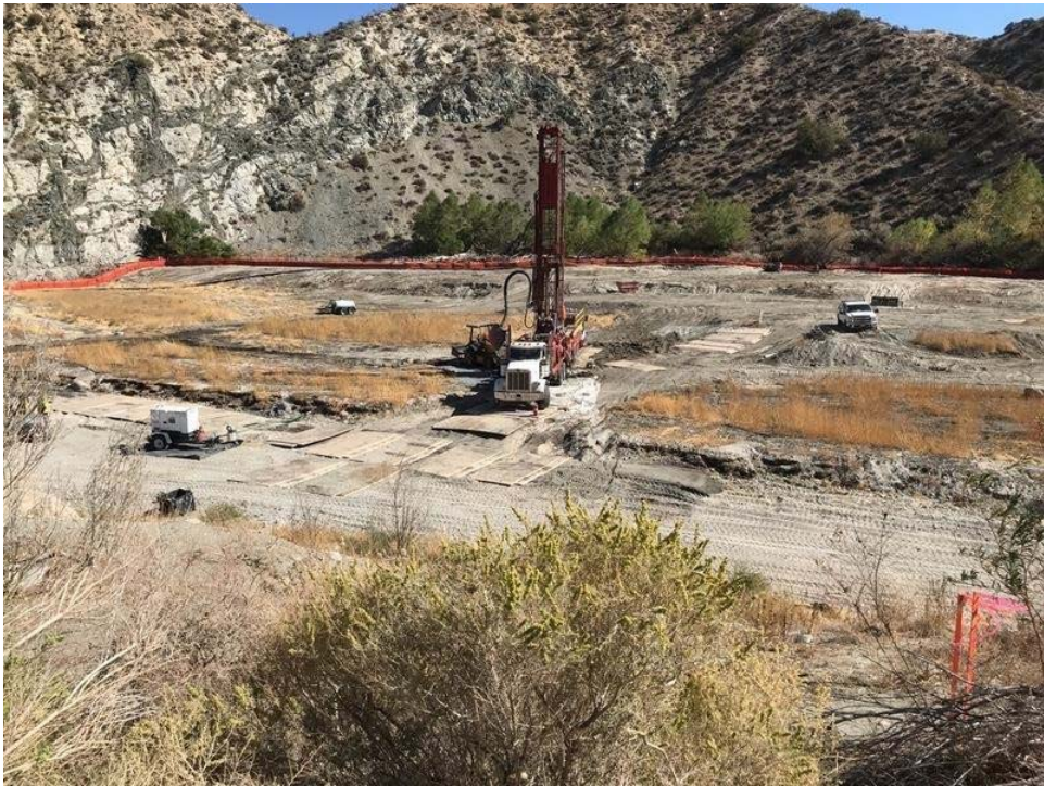
Photo 1. Drilling a dewatering well (October 30, 2018).
