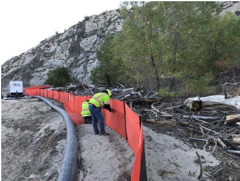
Photo 4. Ongoing maintenance (November 9, 2018).
