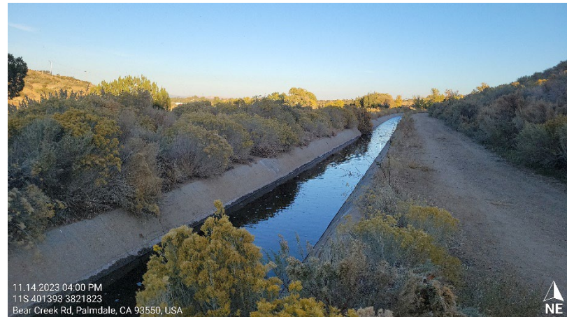
Photograph 4. View northeast of Palmdale Ditch near Bear Creek Road undercrossing.
