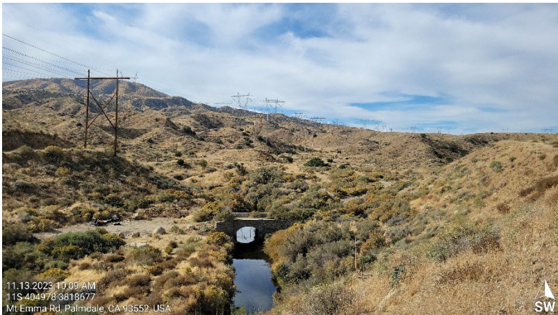
Photograph 3. View southwest of Palmdale Ditch, immediately south of the Mt. Emma Road undercrossing.
