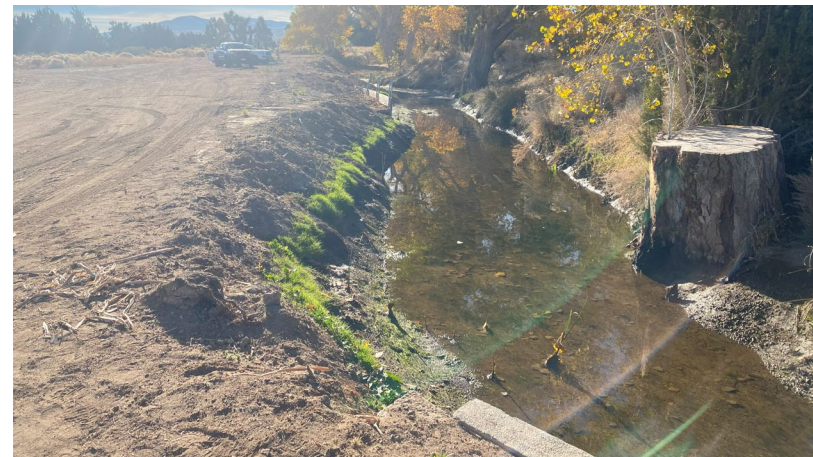
Photograph 4. View south of Palmdale Ditch approximately 240 feet north of Lake Palmdale.
