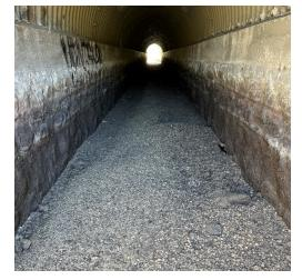
Photo 17: Looking downstream along Tunnel 3 beneath Mt. Emma Road. The tunnel consists of vertical stone and concrete walls supporting a CMP archway. The tunnel has significant sediment accumulation.
