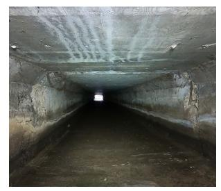
Photo 4-17: Significant concrete loss on both sides of the culvert at this location.
