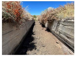
Photo 12: Looking downstream along vertical concrete U-channel with moderate debris along the bottom of the Ditch
