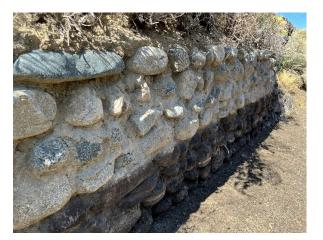
Photo 9: Close-up of vertical cobble/mortar wall
