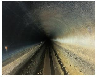
Photo 4-10: Coal tar liner discoloration is more prominent on the west (right) side of the pipe compared to the east (left) side.
