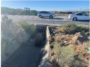
Photo 50: Upstream end of the Pearblossom crossing. Minimal existing cover likely requires a new deeper crossing to be constructed.
