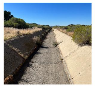
Photo 39: Looking downstream along the trapezoidal concrete-lined channel north of E. Barrel Springs Road.
