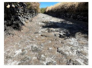
Photo 3: Looking downstream along cobble and mortar section of channel immediately downstream of concrete section
