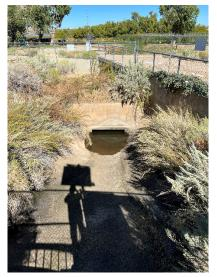
Photo 72: The existing concrete culvert beneath the stormwater channel downstream of the metering flume will remain in place and is not included in this Project.
