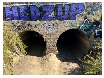
Photo 37: Looking upstream at the downstream end of dual CMP culverts approximately 500 southeast of E. Barrel Springs Road.
