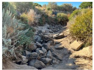
Photo 46: The concrete channel shown in the previous photo transitions to a natural channel as it traverses through a tight curve over large debris.
