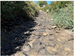
Photo 10: Looking downstream along cobble/mortar Ditch invert
