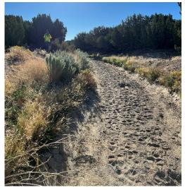
Photo 54: Much of the Ditch in this section has a fine-grained sandy bottom with no concrete lining and moderate vegetation.
