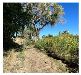
Photo 69: The Ditch downstream of the existing pipe discharge location is curvilinear, overgrown, and undersized to convey a desired flow of 60 cfs.
