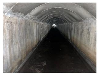
Photo 13: Looking downstream inside Tunnel 1. The tunnel has negligible debris, and the concrete appears to be in good condition.
