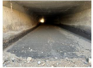
Photo 49: The crossing beneath Pearblossom Highway is an existing concrete box that is not anticipated to be sufficient to convey the required 60 cfs and will be replaced with a deeper, larger undercrossing.
