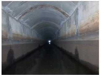
Photo 75: Previous concrete patching, joint weeping, and partially exposed metal in the roof.
