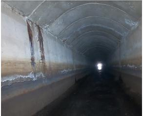
Photo 76: Side wall staining and surface corrosion from joint infiltration
