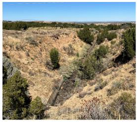
Photo 22: Looking downstream from above the outlet of the 48-inch diameter pipe. The pipe discharges into the deepest section of the Ditch.
