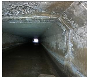
Photo 4-18: Exposed aggregate on the right wall and roof.
