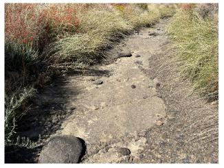
Photo 26: Some sections show evidence along the bottom of the Ditch of possibly requiring rock excavation or increasing bedding depths to install the pipe in the bottom of the Ditch.
