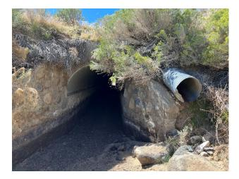
Photo 19: Road drainage from Mt. Emma Road is currently discharging into the Ditch via the pipe shown to the right of the Mt. Emma Road undercrossing.
