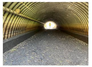
Photo 5: Looking downstream along CMP arch culvert beneath Cheseboro Road
