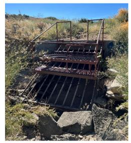
Photo 65: Upstream end of box culvert beneath MetroLink rail tracks.
