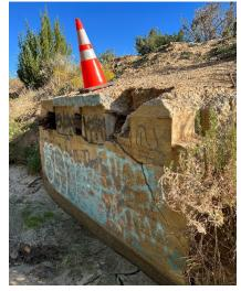
Photo 58: North side of the existing Ditch where old concrete bridge abutments exist.
