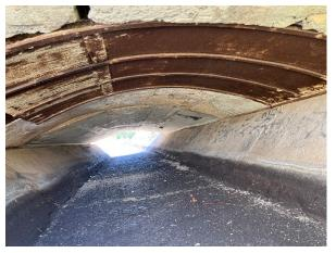
Photo 28: There is one steel/concrete bridge over the Ditch approximately 440 feet from 47th Street East. This bridge does not provide sufficient capacity to convey 60 cfs and will need to be removed as part of the Project.
