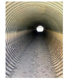
Photo 38: Looking upstream at the inside of one of the CMP culverts shown in Photo 37.
