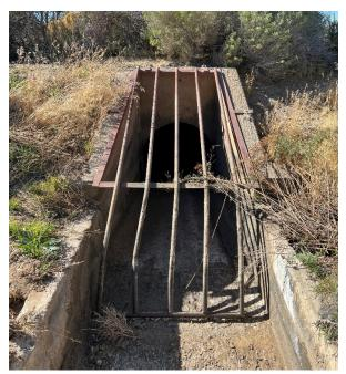
Photo 41: Upstream end of buried 36-inch diameter RCP pipeline that crosses the State Aqueduct as an aerial 36-inch steel pipe.
