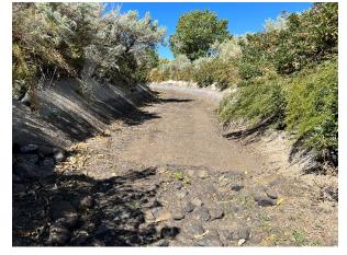
Photo 11: Transition from mortar/cobble to concrete lining
