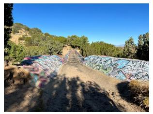
Photo 55: Looking downstream along the existing steel flume. The flume will be demolished as part of the Project and replaced with a buried siphon.
