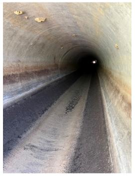
Photo 30: Looking upstream inside the 48-inch RCP culvert beneath 47th Street East.
