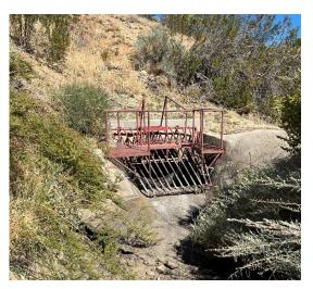
Photo 20: Existing trash rack on the upstream side of the existing 48-inch diameter pipe just north of Mt. Emma Road
