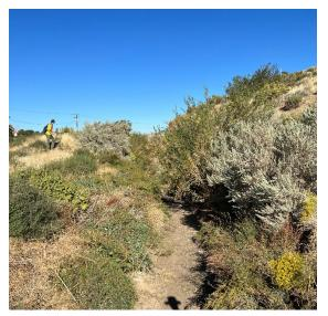
Photo 64: Looking upstream at the native earthen Ditch within MetroLink's right-of-way. Steep slopes from the east (right) prevent installing the new pipeline outside of MetroLink right-of-way.
