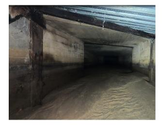
Photo 4-13: Looking upstream. Masonry/metal channel transitions to a cast-in-place concrete box beneath Sierra Highway.
