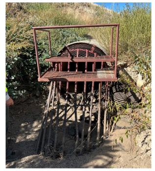
Photo 29: Looking downstream at the 48-inch RCP culvert beneath 47 Street East. It is anticipated that this trash rack will be removed for connection to the new pipeline.
