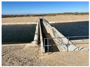
Photo 44: The 36-inch steel pipe is located parallel to the concrete U-channel that conveys stormwater runoff across the State Aqueduct.
