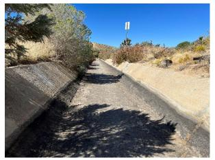
Photo 27: As the Ditch approaches 47th Street East it transitions to a trapezoidal lined concrete channel.
