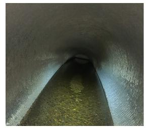
Photo 4-9: Sand and pebbles can be seen beneath the water at the existing sag. Mild to moderate rebar exposure is also evident.
