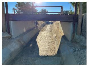
Photo 51: The City has crossed the Ditch in two places with pedestrian bridges that may need to be removed depending on the final pipeline alignment.
