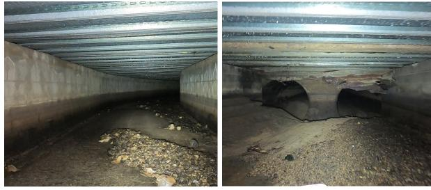
Photo 4-11: Looking downstream at debris. Note the vertical masonry sidewalls and metal roof.
