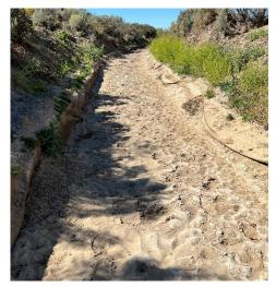
Photo 36: The Ditch transitions to a sandy bottom underlain by a geotextile fabric as it approaches E. Barrel Springs Road.
