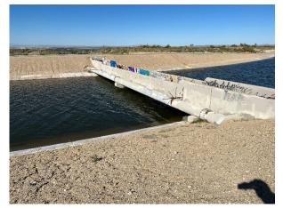
Photo 43: 36-inch steel pipe crossing the State Aqueduct
