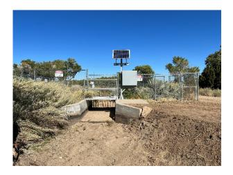
Photo 71: The existing metering flume at Lake Palmdale is undersized to handle the ultimate flow rate of 60 cfs and will need to be replaced as part of this Project.
