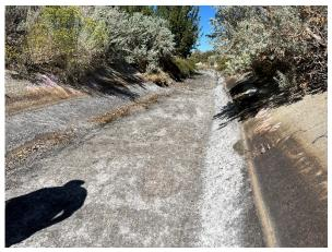
Photo 4: Looking downstream at concrete repair section within cobble/mortar section
