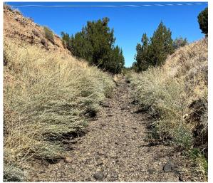
Photo 23: This section of the channel has varying gradations of soil and rock along the bottom. Moderate rocks/cobbles shown here.
