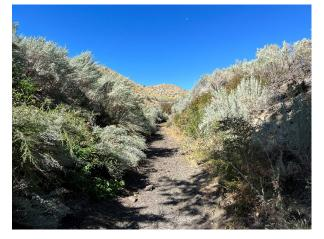
Photo 7: Looking downstream along overgrown channel with native soil bottom downstream of Cheseboro Road
