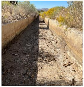
Photo 40: Looking downstream as the Ditch transitions to a narrow concrete U-channel with vertical walls. It is anticipated this channel will be demolished to install the new pipe.
