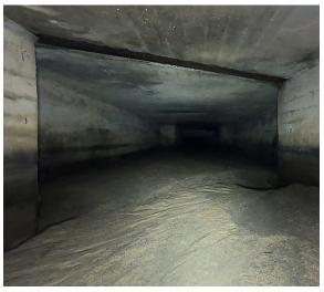
Photo 4-14: The concrete box expands and deepens. This box is filled with approximately 24 inches of sand.
