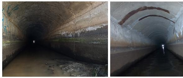
Photo 73: Downstream end of Tunnel #2. Debris and highwater mark is visible.
