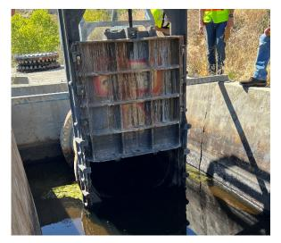
Photo 1: Existing slide gate at the upstream limit of the Project
