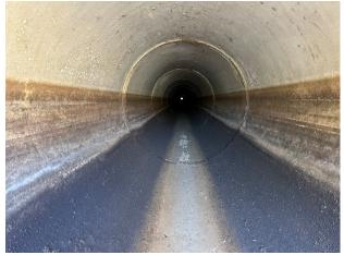
Photo 21: Looking upstream at the existing 48-inch diameter pipe, referenced in Photo 20
