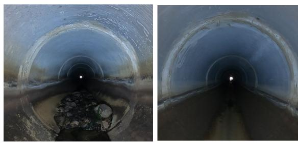
Photo 79: A pile of rocks is present within the pipeline and needs to be removed during construction.
