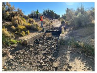
Photo 52: Looking upstream at the easterly drop structure along this segment.
