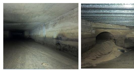
Photo 4-15: Looking upstream. The AVEK tie-in beneath Sierra Highway can be seen on the right wall. Per as-builts, this pipe was installed with the invert 24 inches above the floor of the culvert, but is now in danger of being blocked by sand.
